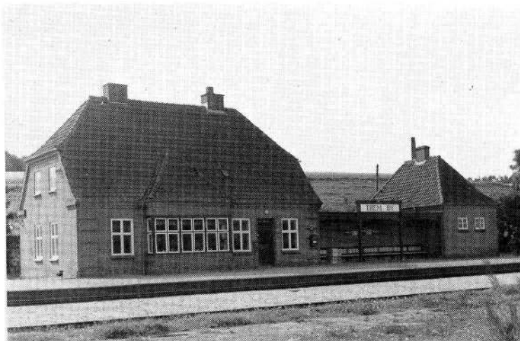
HBS, Them By stationsbygning, perronside
