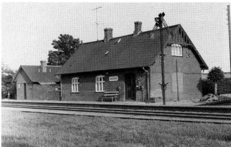
HBS, Vestbirk, 1964 (hol) stationsbygning, perronside
