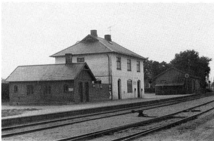
HBS, Østbirk, 1964 (hol) stationsbygning, perronside
